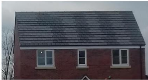
Figure 8. Example of concrete roof tiles exhibiting efflorescence (on left) and then after 3 years of natural weathering
