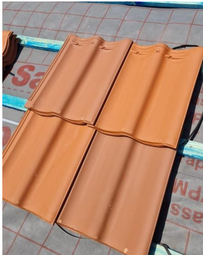
Figure 10. Example of natural colour variation in fired clay roof tiles
