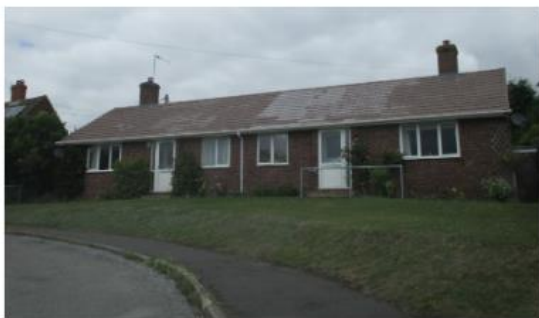
Figure 9. Example of concrete roof tiles exhibiting efflorescence (on left) and then after 4 years of natural weathering
